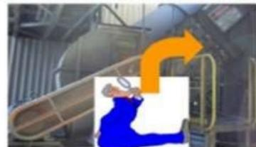
Figure 1 - Exhauster's damper to adjust the volumetric air flowrate of the baghouse.
