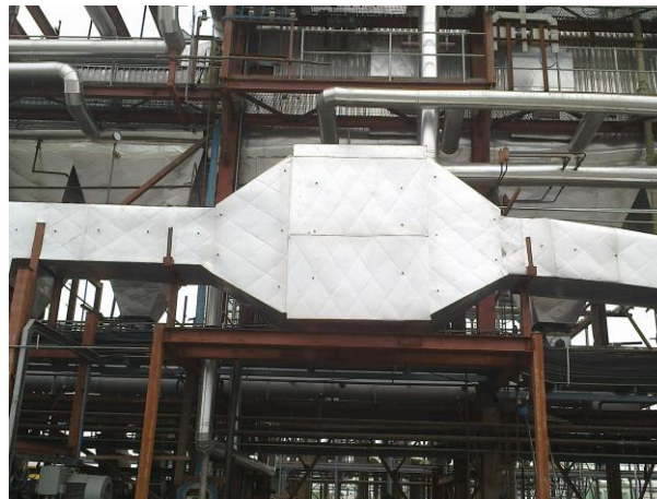
Steam Coil Air Pre Heater (SCAPH)
